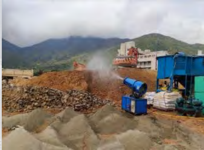
Water spraying via mist cannon at the idled construction materials
