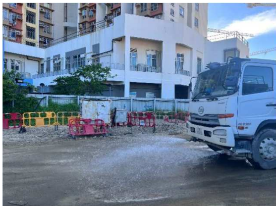
Water spraying by water truck for dust control
