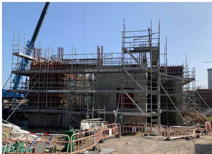
RC Structure and E&M Works for Pumping Station in progress
