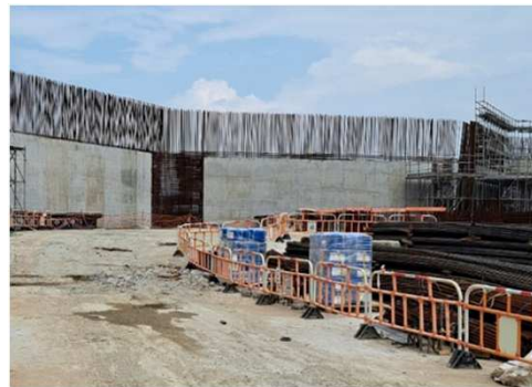
Rebar fixing of wall of service reservoir
