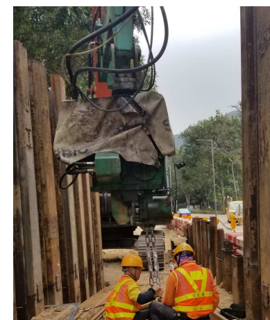
Noise mitigation measures on sheet piling works
