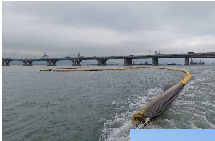
Maintenance of perimeter silt curtain (All silt curtain removed in Mid-August 2023)
