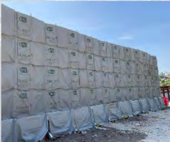
Deployment of noise barrier
