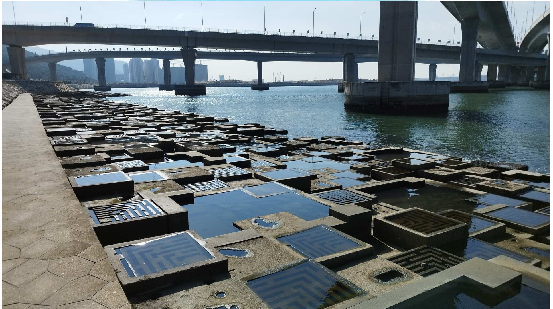
General View of Rocky Eco-shoreline
