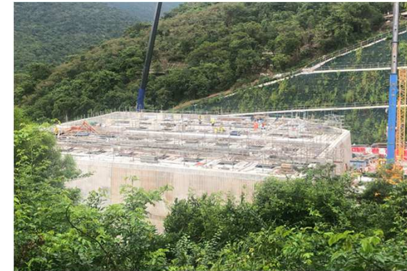
Salt Water Service Reservoir
