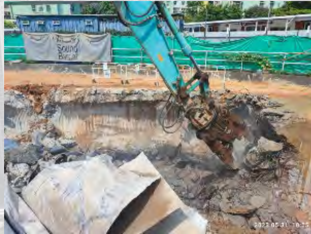
Demolition activity by silenced type Powered Mechanical Equipment (PMEs)
