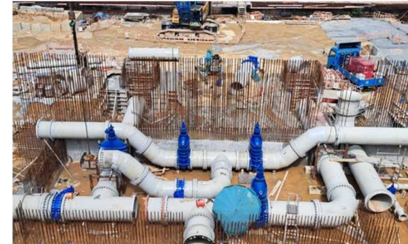
Installation of watermain in valve chamber
