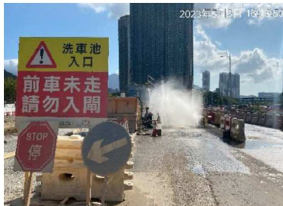
Wheel washing bay with high pressure jet
