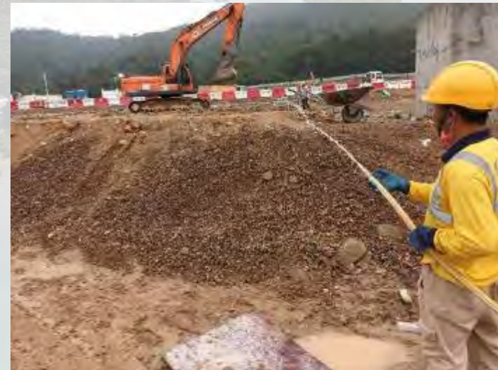
Water spraying by manual hose during materials handling
